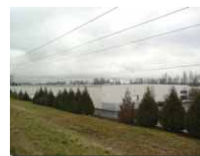
BUILDING SCREEN EXAMPLE 3
