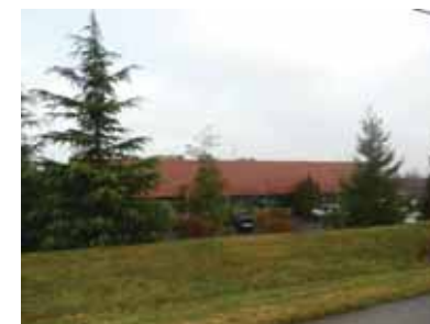
BUILDING SCREEN EXAMPLE 2
